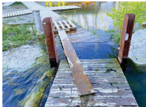
APSC dock and beach area flooded, May 22.
